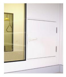
These elements had been designed to make easy the access to the technical elements located behind partitions
