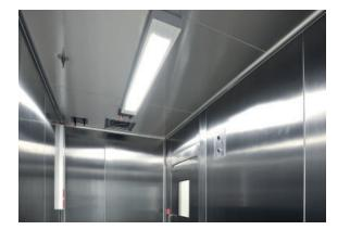
The Stainless steel coving sections are designed for the sanitary cladding of partition-to-partition and partition-to-ceiling angles. Their rounded shape facilitates the cleaning according to the hygiene rules.
