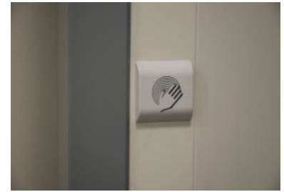
control by 2 proximity detectors (1 each side)
