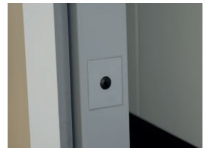
2 rows of horizontal safety photocells
